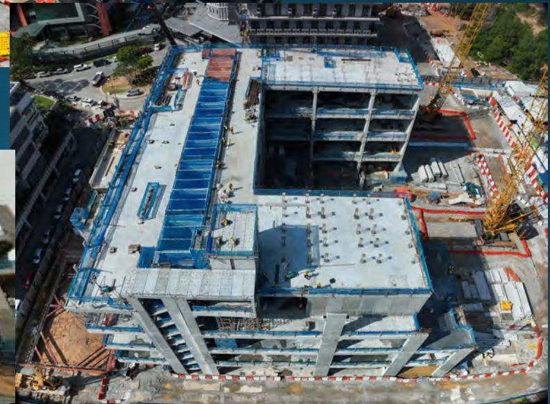
Precast Installation & Topping Slab
