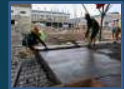
Concrete Casting & Levelling
